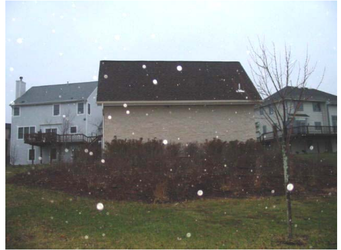
6 th Hole Pump House
